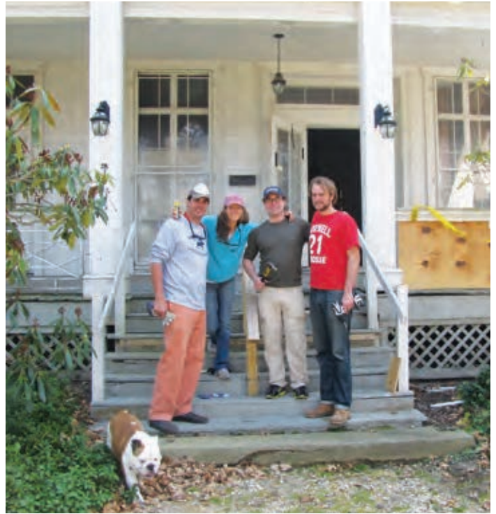
Young members helped with repairs at the Trousell House in Oyster Bay
