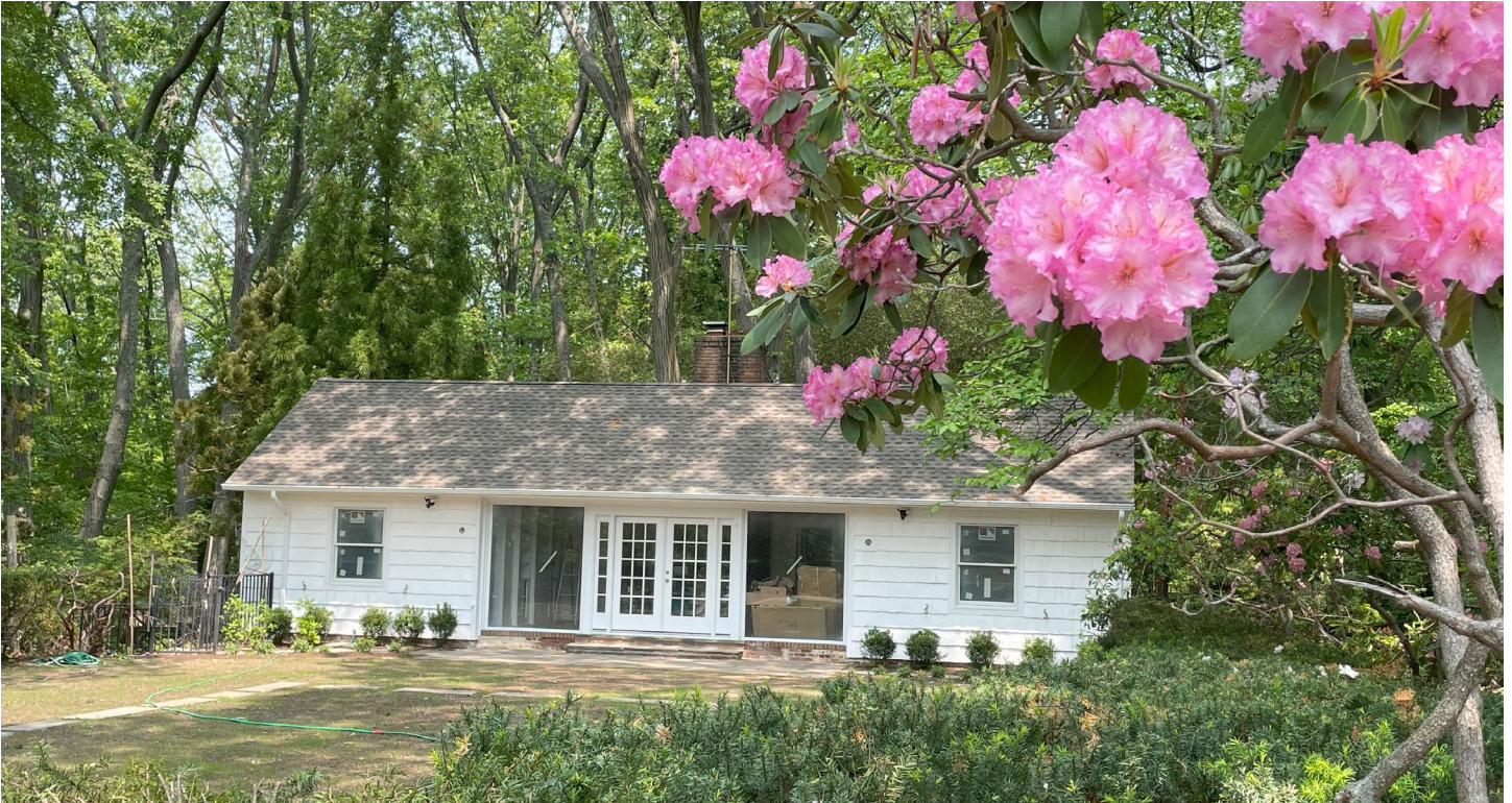
The Margaret K. Sullivan Education Annex at the Humes Preserve will be used to host classes, lectures, workshops and events. It opened on June 15th with a native plant sale and lecture.
